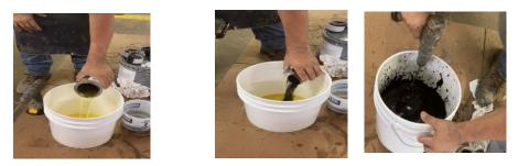
2. Pour part A into the part B and pigment and mix for one minute.
