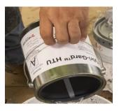
3. Pour part C aluminum oxide into bucket and mix for another minute
